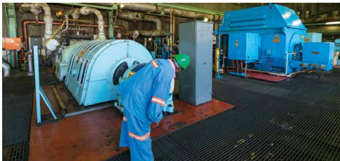
Power Plant turbine units
