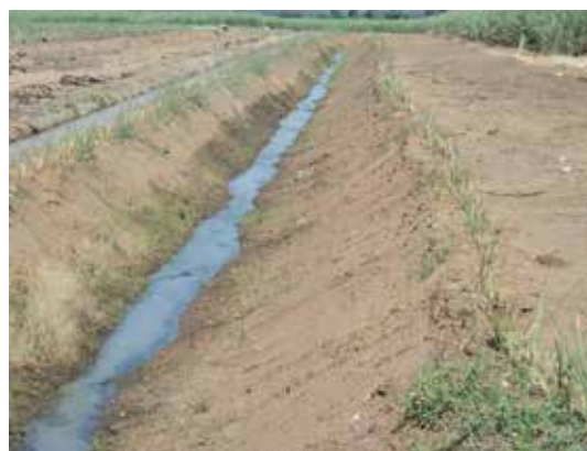
Newly planted Vetiver grass on a recently maintained field drain
