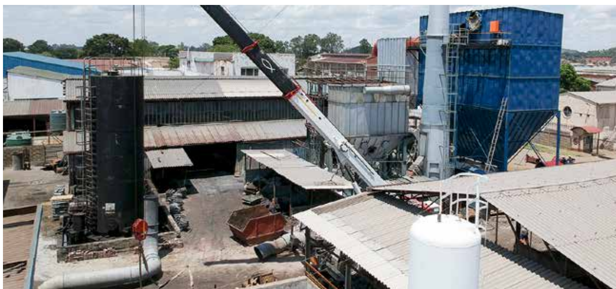
Installation work of a new filtration plant at the batteries division
