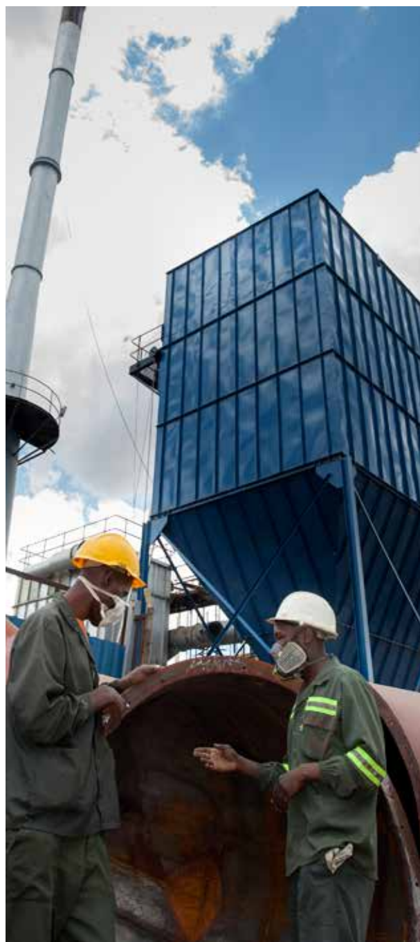
Installation work of a new filtration plant at the batteries division
