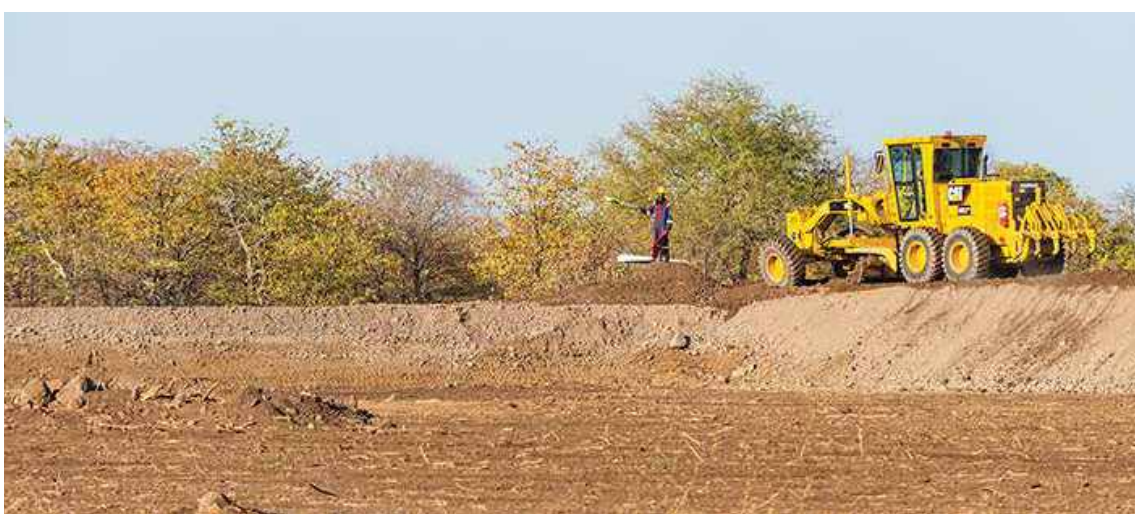
Overnight storage dam construction
