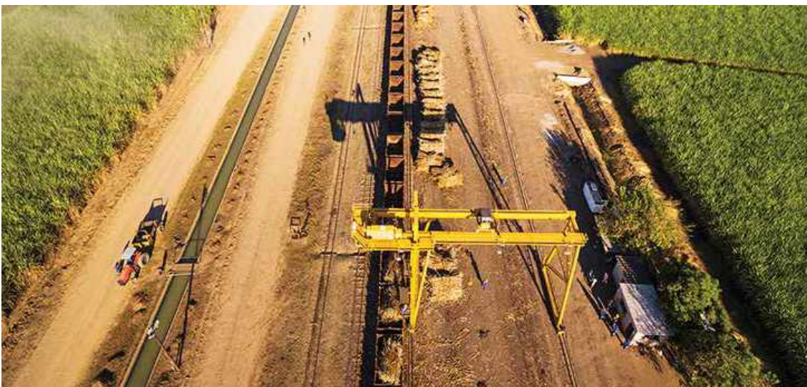
Rail loading zone
