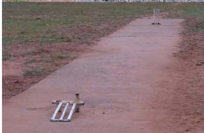
Above: We also donated quarry stone for a Cricket Pitch at Mosi-oa-Tunya High School
