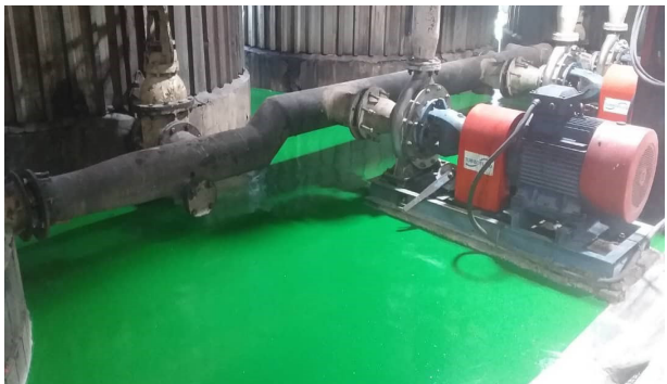
Epoxy floor at Hippo Valley Mill.
