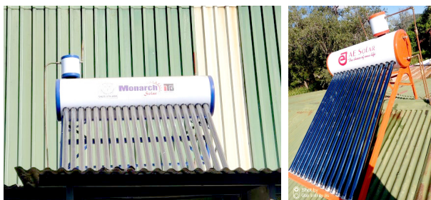
Replacing electric geysers with solar geysers
