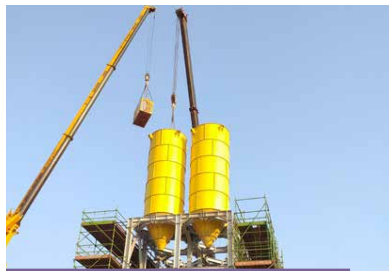
Silo positioning works during the installation of the new Dry Mortars Plant.
