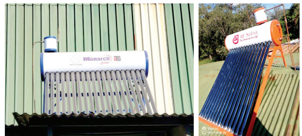
Replacing electric geysers with solar geysers
