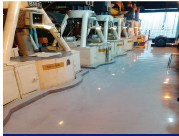
Epoxy floor at Hippo Valley Mill.
