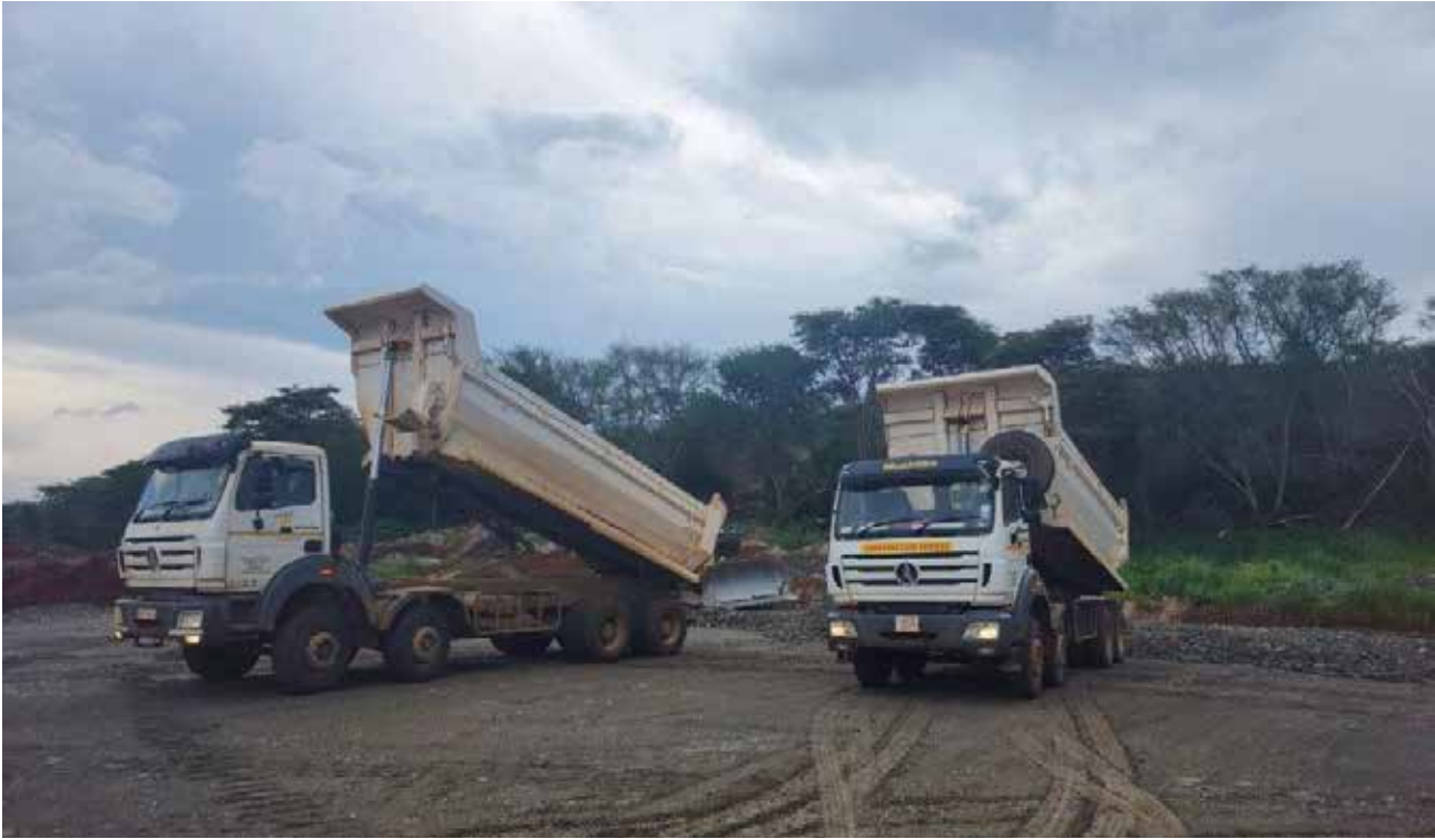
Hauling waste rock material to build the Starter Wall
