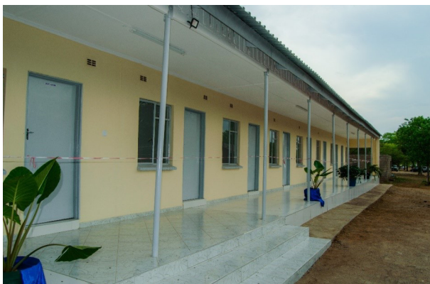
The Zimbabwe Republic Police 12-Office Block constructed to provide space for 60 officers.
