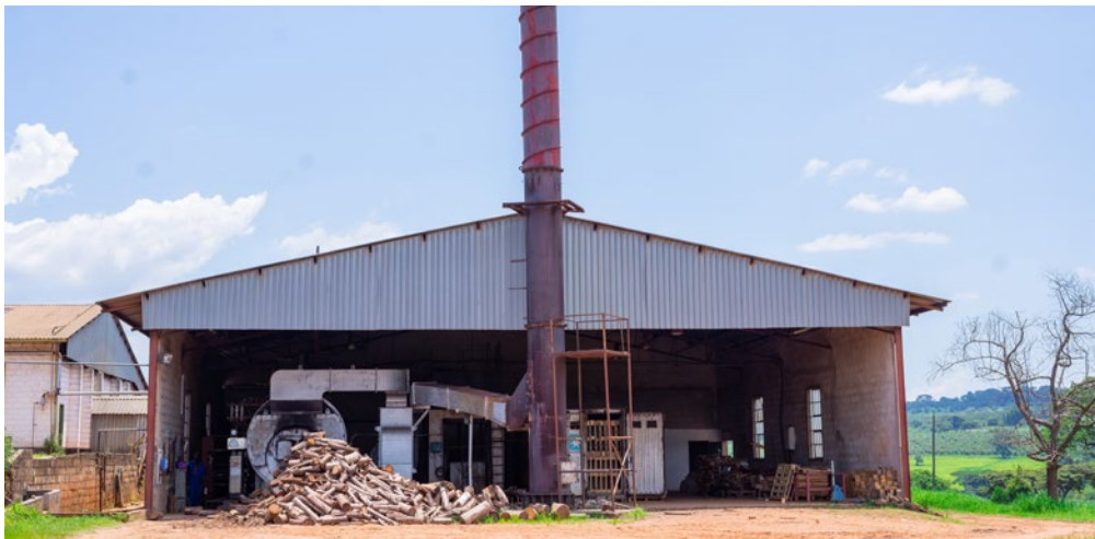
Boiler chimney on the Zona tea factory
