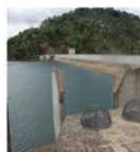
Tugwi-Mukosi Dam Level - 100.0%
